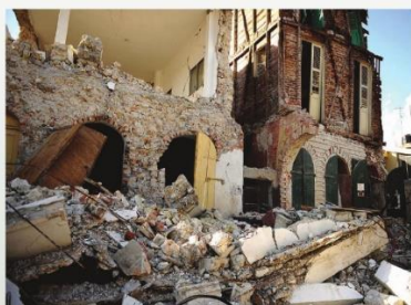
► THE BUILDING IN THE FOREGROUND SUFFERED MORE DAMAGE THAN THE BUILDING IN THE BACKGROUND AFTER THE 2010 EARTHQUAKE IN HAITI. WHAT FACTORS COULD EXPLAIN THIS? PHOTO BY THE PHOTOS BY HURUP, GETTY IMAGES
