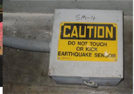
▶ SENSORS WILL RECORD ANY VIBRATIONS, INCLUDING THOSE NOT CAUSED BY EARTHQUAKES.
